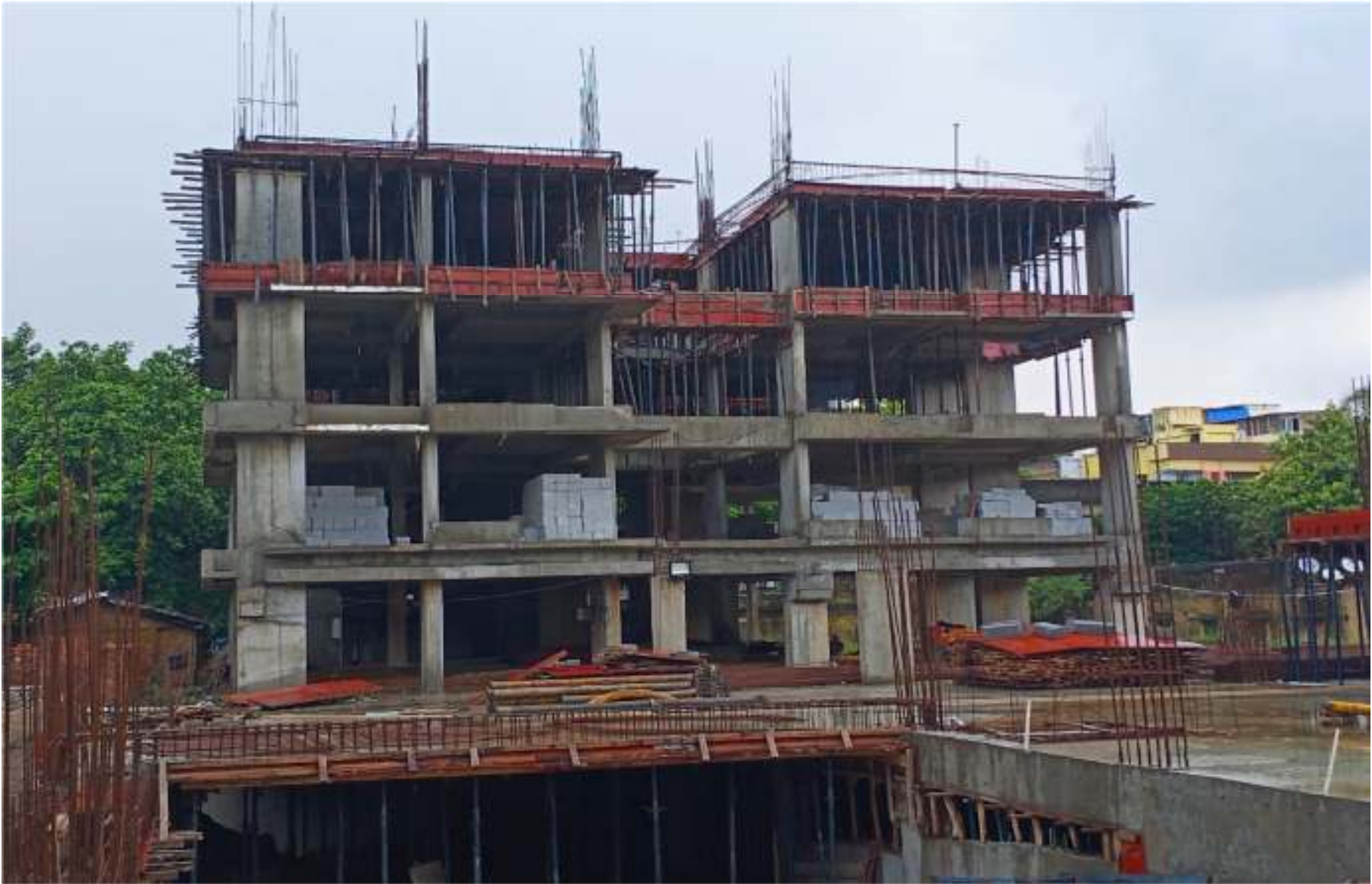
BLOCK 2, 4th floor shuttering wip
