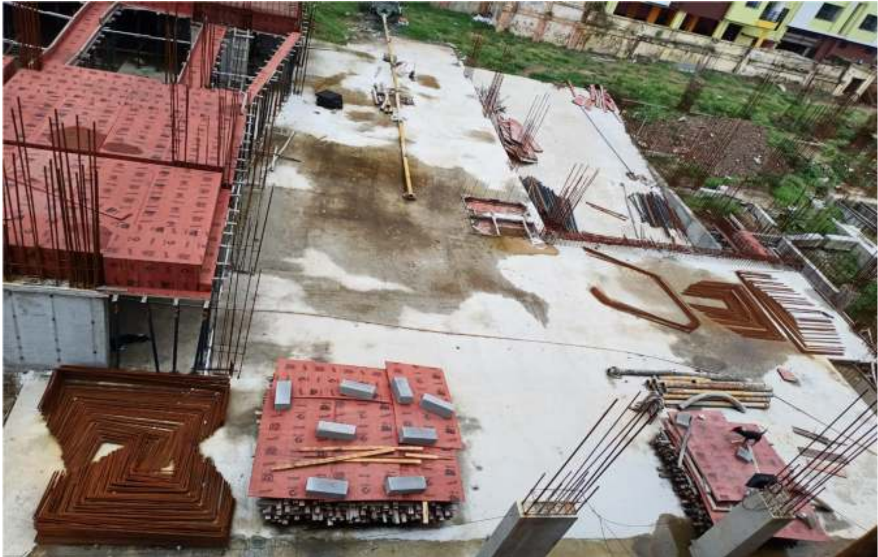
Podium top slab including Ramp casting completed.
